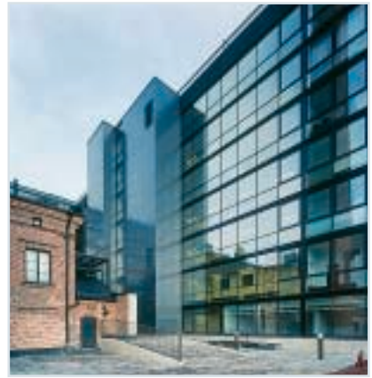
As Oy Helsingin Bulevardinaukio, Helsinki PK 103, 400 x 1500 mm, 1.2 mm, Pvdf RR23, yht. 900 m 2
